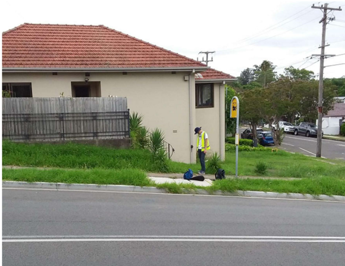
Figure 4: Example of a bus stop in the City of Ryde LGA with steep end-fall (Image source: City of Ryde Council)
